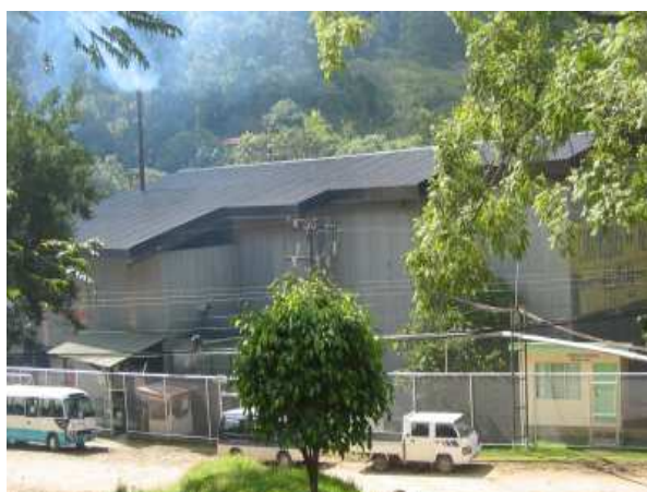
Figure 7: Coffee drying, Coopeldos, Costa Rica. Installed capacity: 595 kW th (850 m 2 Solar Wall ® collector)
